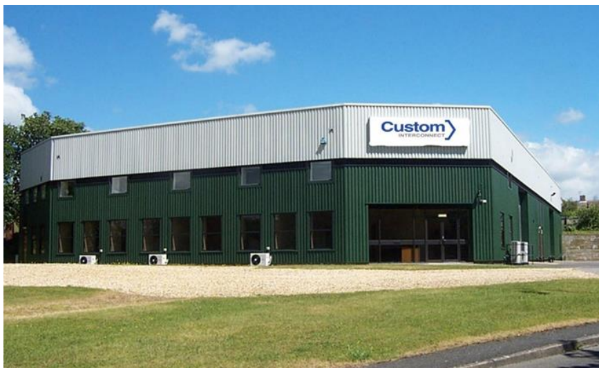
CIL House – 24,000sq ft Prototype manufacture + Small to Medium volume PCBA production
